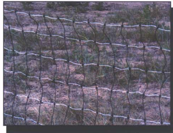
Figure 3b—Unless this fence is kept tight, the flexible vertical strands may allow hot wires to sag, shorting out the fence.
